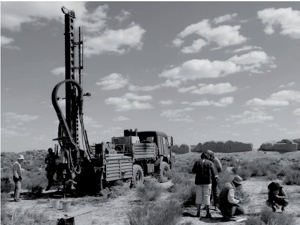
Fig. 6. Mechanical coring in the interior of Dzhankent in 2019
